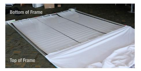
Step 9. Feed the power cables from the Brite Panels through the wire management holes in the white fabric back of the graphic.
